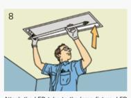
Attach the LED tube to the lamp fixture. LED tubes can be attached in either directions.
