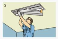
Dismantle lamp fixture to replace the ballas stabilizer.
